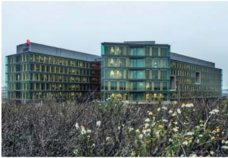
Head office PriceWaterhouseCoopers, Gasperich, Luxemburg BREEAM Very Good / Completion 2014 ETAP solution with UT1 recessed luminaires, R8 and R4 mounted luminaires and E6 industrial luminaires.
