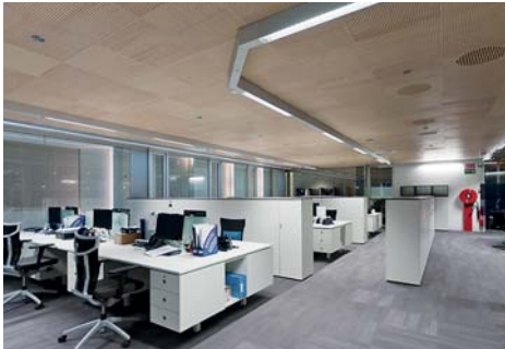
Regional head office Naturgas Energía, Bilbao, Spain LEED Platinum / Completion 2013 ETAP solution with Kardó modular light lines and D42 LED downlights
