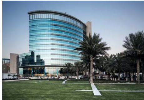
Headquarters Majid Al Futaim, Dubai, United Arab Emirates LEED Gold / Completion 2014 ETAP solution with Flare spots, D42 downlights, R7 suspended luminaires with occupancy detection and U7 recessed luminaires (all LED)
